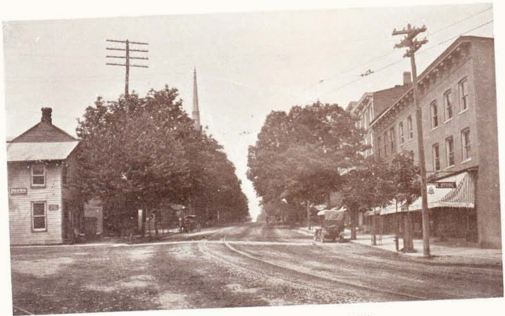
MAIN STREET—Looking West From Above Fifth
